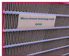
Aluminium micro channel heat exchanger
